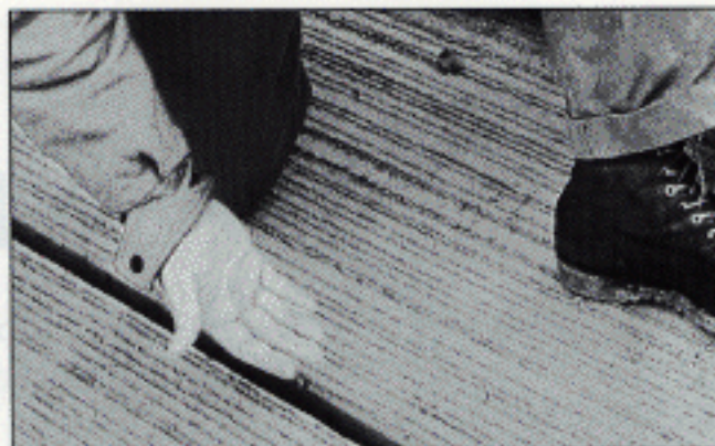
Figure 3. Dirt and dust on the reservoir sidewalls will inhibit bonding of the sealant. If you find any traces of contamination, reclean the joint.
