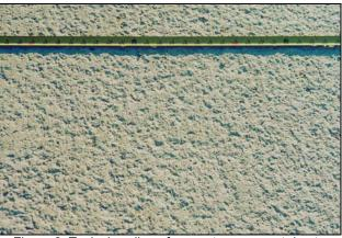
Figure 2. Typical scaling of concrete pavement due to non-durable paste on surface.
