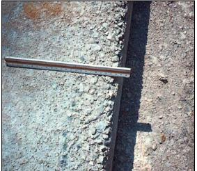
Figure 5. Edge erosion of freshly-placed slab due to rain.
