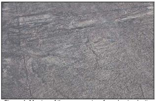
Figure 1. Marring of the pavement surface due to plastic sheeting. Does not require remediation unless ride quality or skid resistance is unduly affected.
