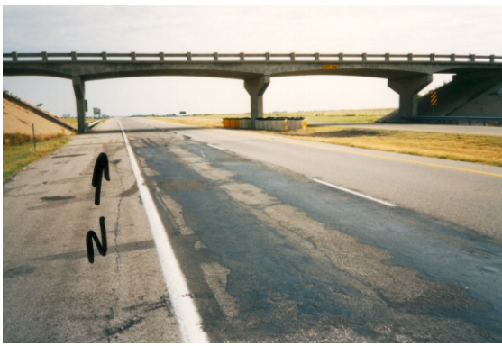
100-mm asphalt overlay on rubblized JRCP
