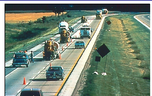
Diamond Grinding of an old concrete pavement to restore smoothness
