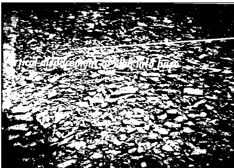
Rubblized concrete pavement. Note the lack of uniformity in the rubblized material. 16
