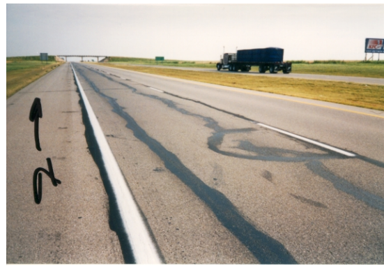
200-mm asphalt overlay on rubblized JRCP
