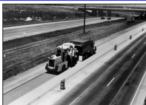
Shotblasting the surface in preparation for a bonded concrete overlay.
